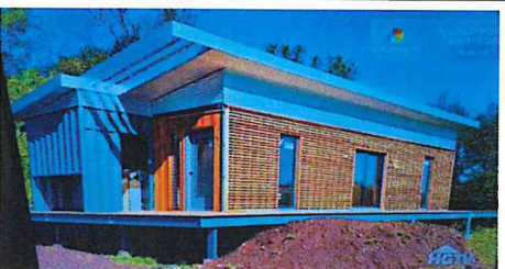
Horizontal wood slat exterior cover
